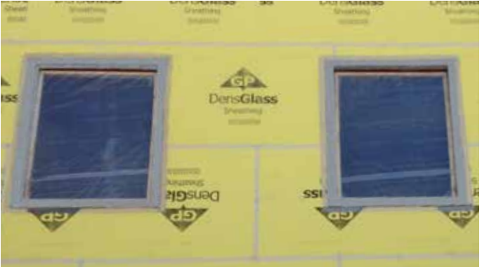
Seams detailed with CLIMATE FLASH™ Flashing Tape
