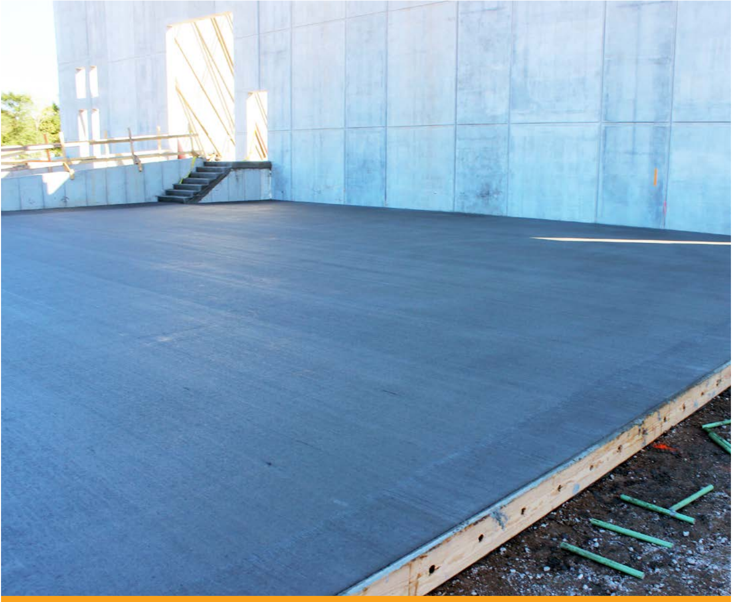
A freshly placed and finished concrete slab
